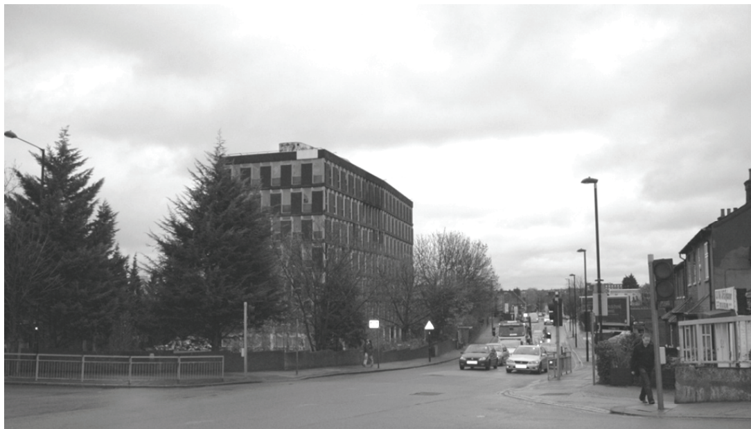
Existing Site Photo
